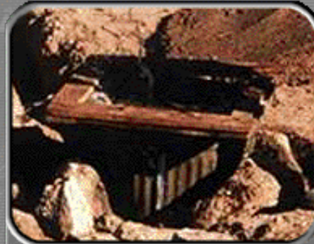
Barrel filter grease trap
