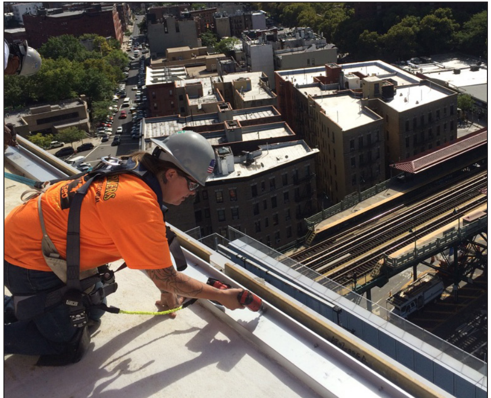
Tamara Gabbard working at 125th and Broadway in Manhattan, finishing 11th floor curtain wall covers. She is employed with Enclose contractors through the Local 580 Ironworkers Union as a first year apprentice.
