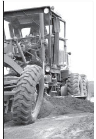
Sgt. Patrick McCarthy levels a final coat of topsoil with a grader. Photos by Staff Sgt. Mike R. Smith.
