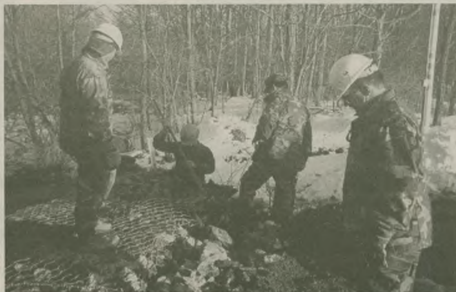
Members of Binghamton's 10th Brigade of the New York Guard work to restore stone-filled berms at the state's Guilderland Range Facility following the devastating rains of Hurricane Floyd. Inset: The State Police target shack was nearly destroyed by floodwaters. Photos by Major John Sacca.
