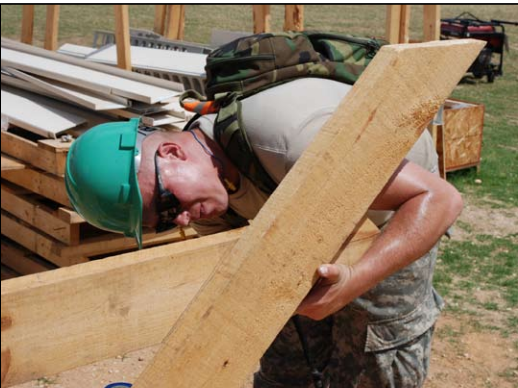
Private First Class James Bach, an engineer with the 1156th Engineer Company, New York Army National Guard finishes a picnic table for the children of St. Mary's orphanage in the town of Tacarigua, Trinidad as part of Operation Beyond the Horizon 2008. The engineers are also building a school and a medical clinic for the children of the orphanage. Photo by Sgt. 1st Class Peter Towse.
