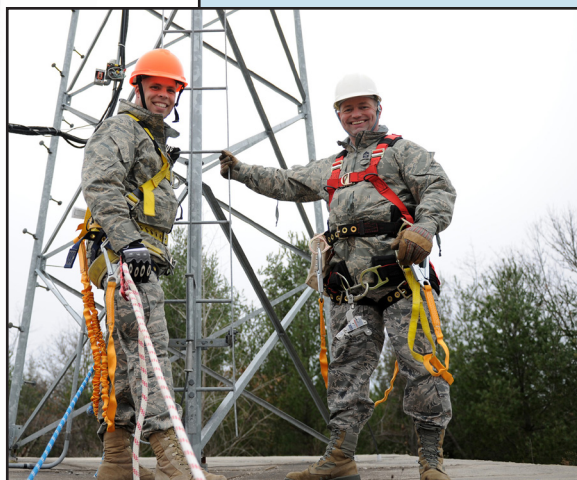
FORT DRUM - New York Air National Guardsmen Chief Master Sgt. Russell Youngs, the 174th Fighter wing's Command Chief and Tech. Sgt. Michael Griepsma prepare to climb an 85-foot communications tower at the Adirondack Range, Fort Drum, on Nov. 22. The towers are used to hold cameras to view targets down range. Photo by Tech Sgt. Ricky Best, 174th Fighter Wing.
