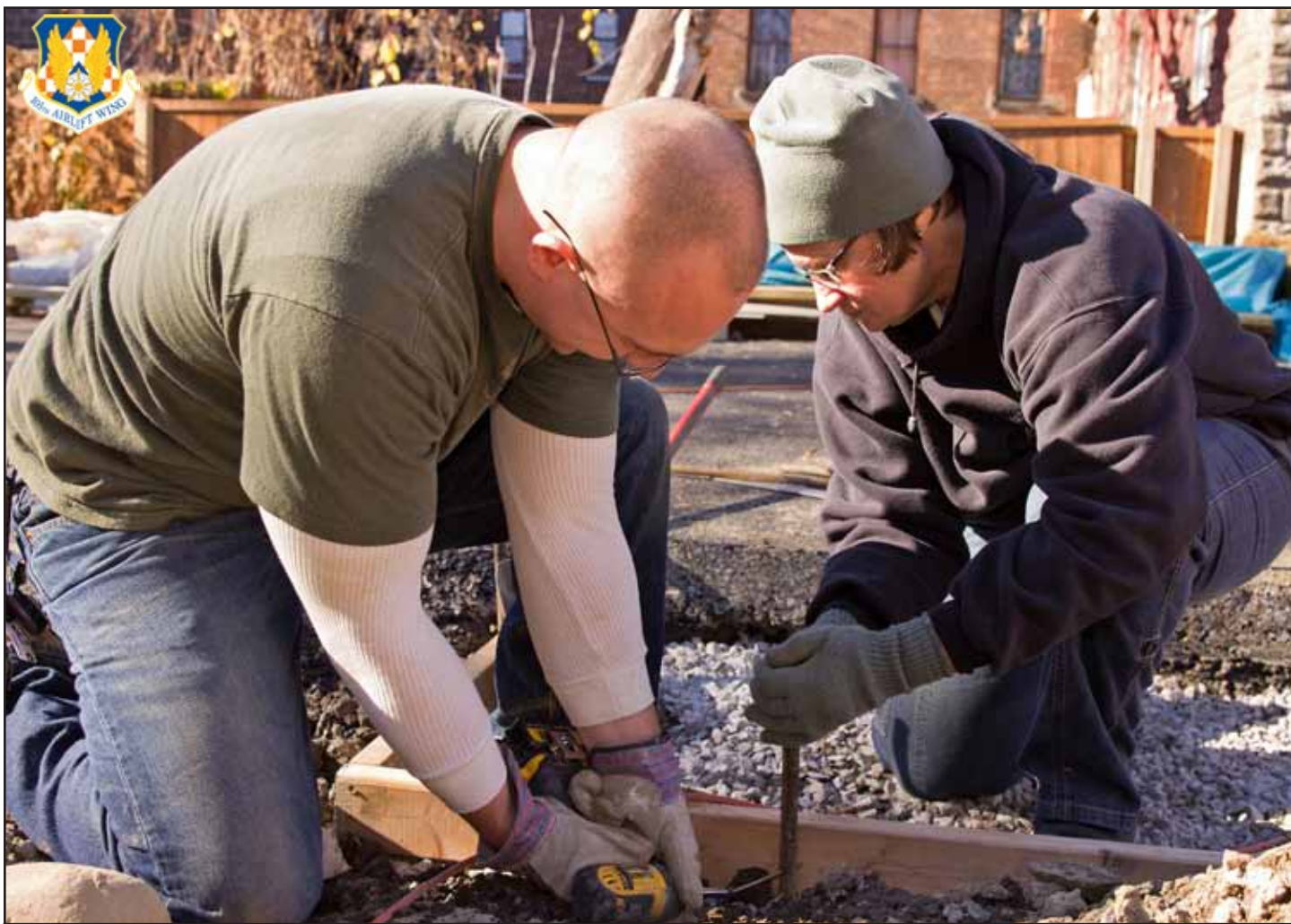
Tech. Sgt. Daniel DiChiara, president of the 105th Airlift Wing First Six Council, uses a cordless drill to drive a screw through a stake and into a wooden board while Senior Master Sgt. Elizabeth Colton, of 105th Logistics Readiness Squadron Aerial Port, holds the stake steady.
