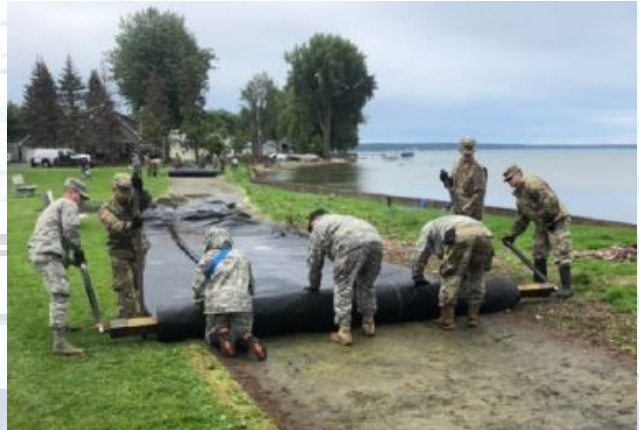
Removal of water bladder at Sackets Harbor
